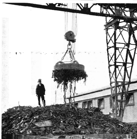
PICTURED HERE is the overhead crane at the Reclamation Depot, Spotswood. It hovers over the twisted mass of iron and steel and picks up two tons at a time by electromagnetic. Since the Depot was created in 1926, the value of materials sold and or issued totals nearly £1,000,000. Under present war time conditions, the Depot is of immense importance.
